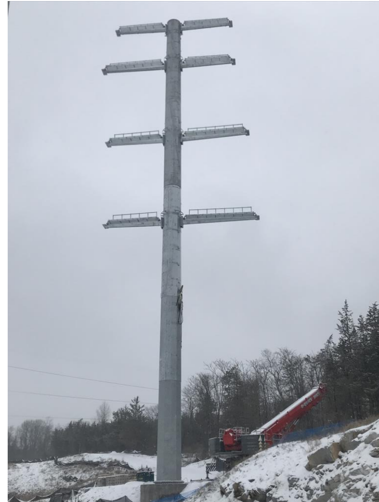
Final Tower Constructed Near CVEC
