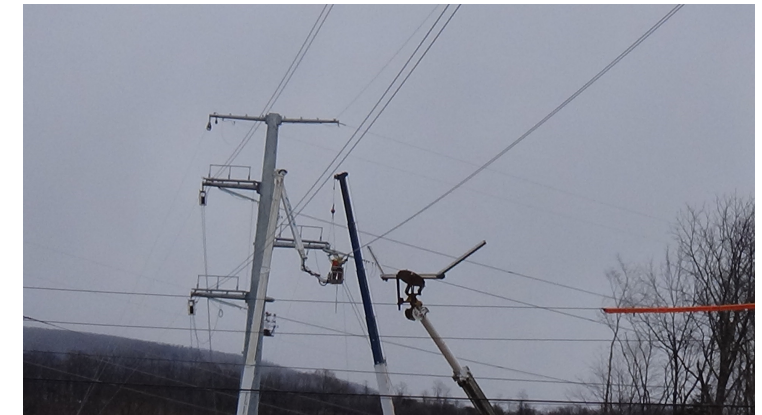
Installing Conductors
