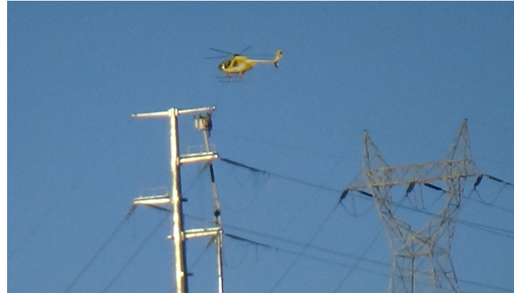
Installing Conductors
