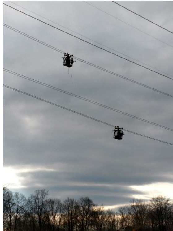
Installing spacers between conductors
