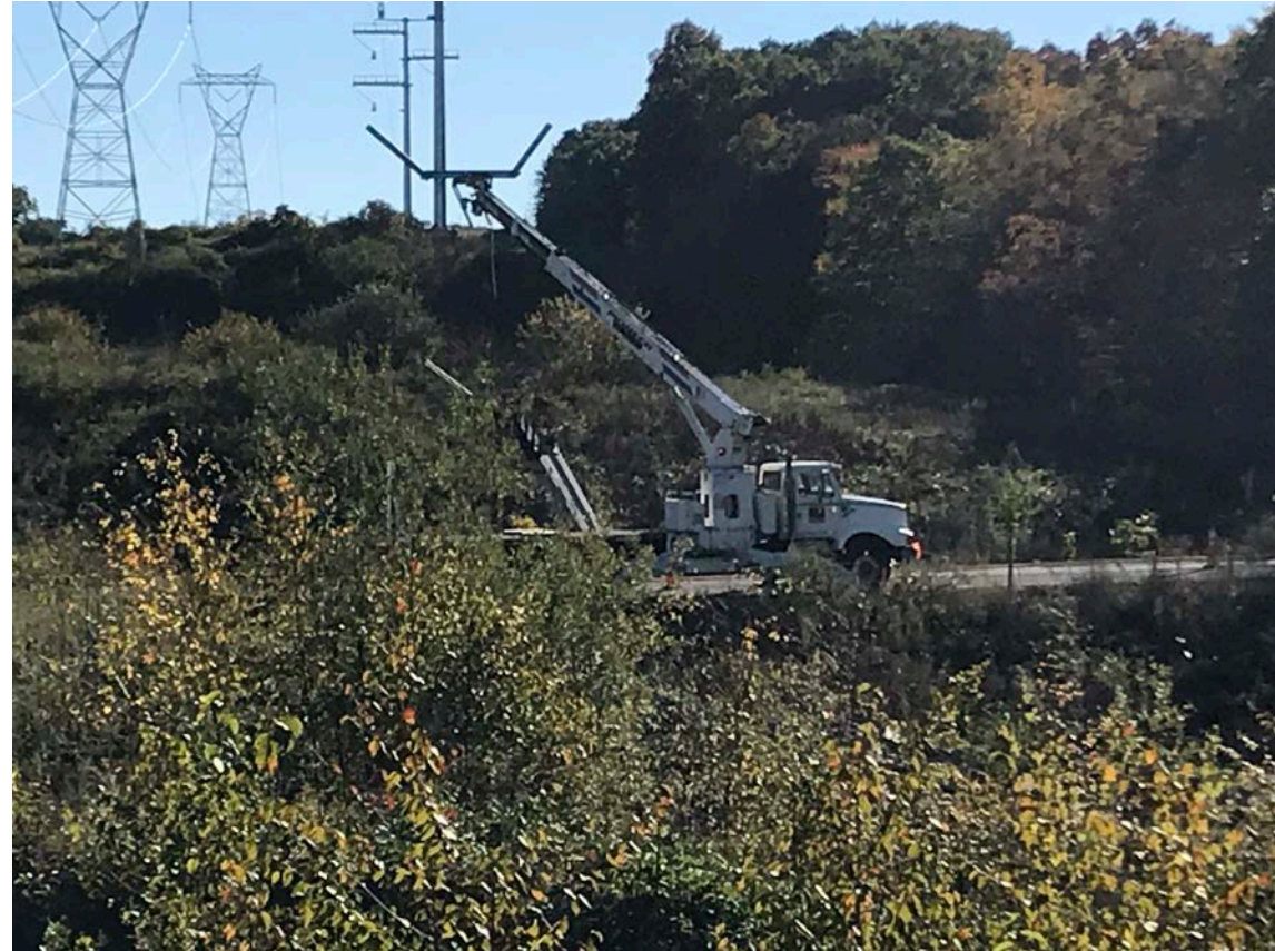
Guard Structure Over Taconic Parkway
