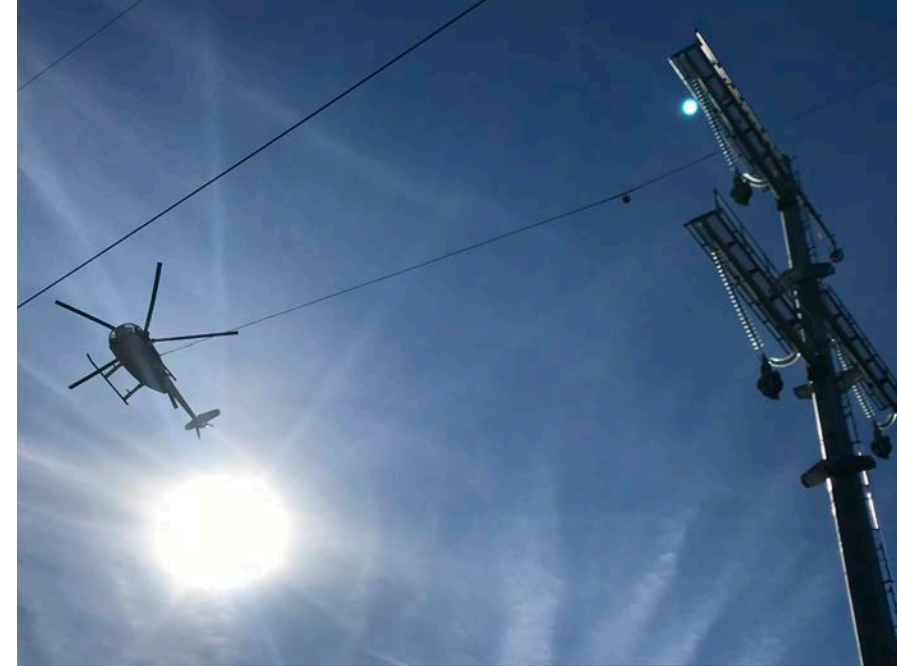
Helicopter Stringing Pull Rope
