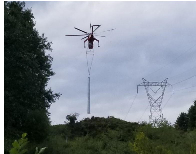
Helicopter Construction of Towers
