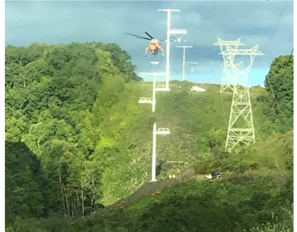
Installation of Top onto Base
