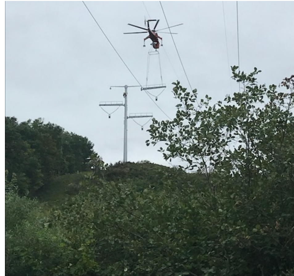
Installation of Conductor Arm
