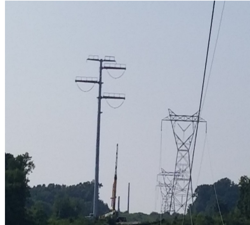
Conductor arms and insulators installed
