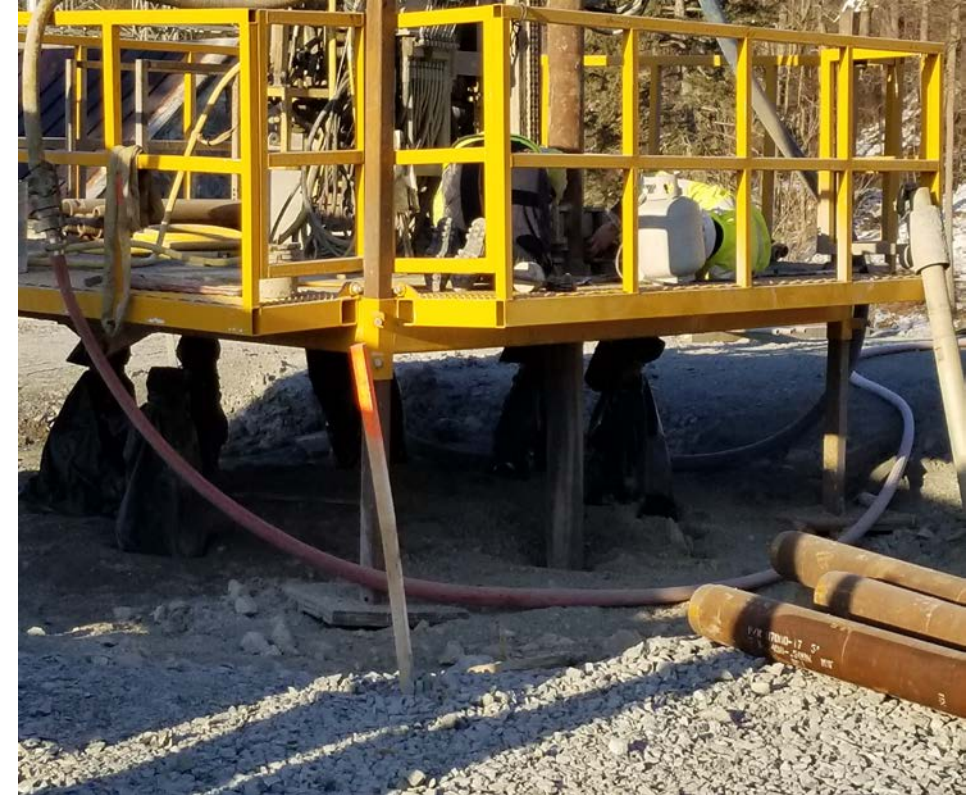
Micropile drilling
