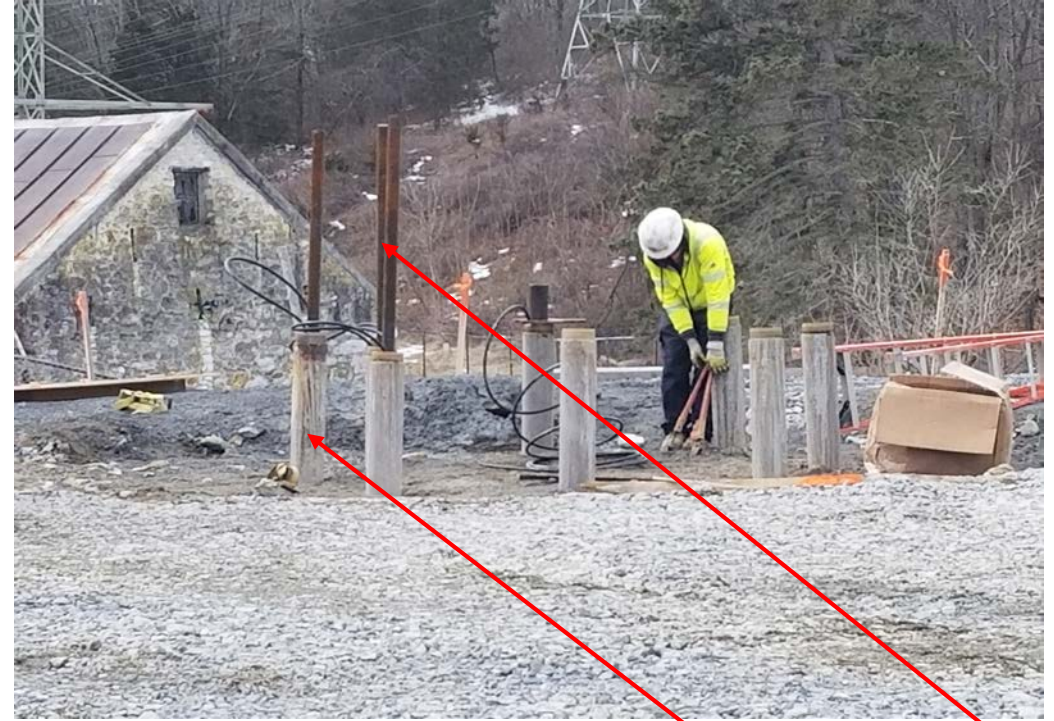
Micropile construction: sleeves and rods
