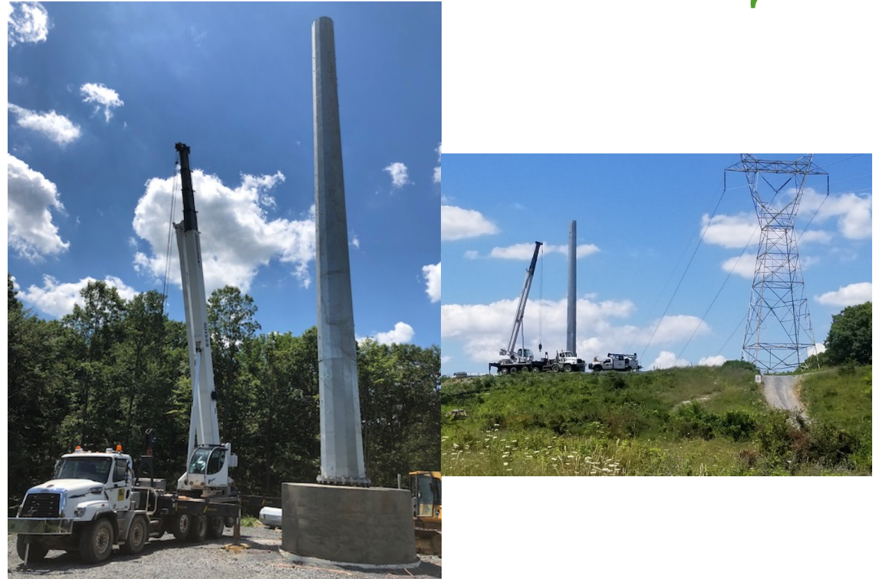
Base and Mid Section of Tower installed
