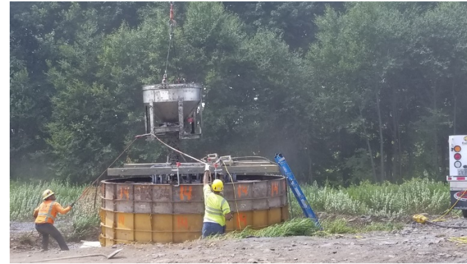
Helicopter Assist Concrete Cap
