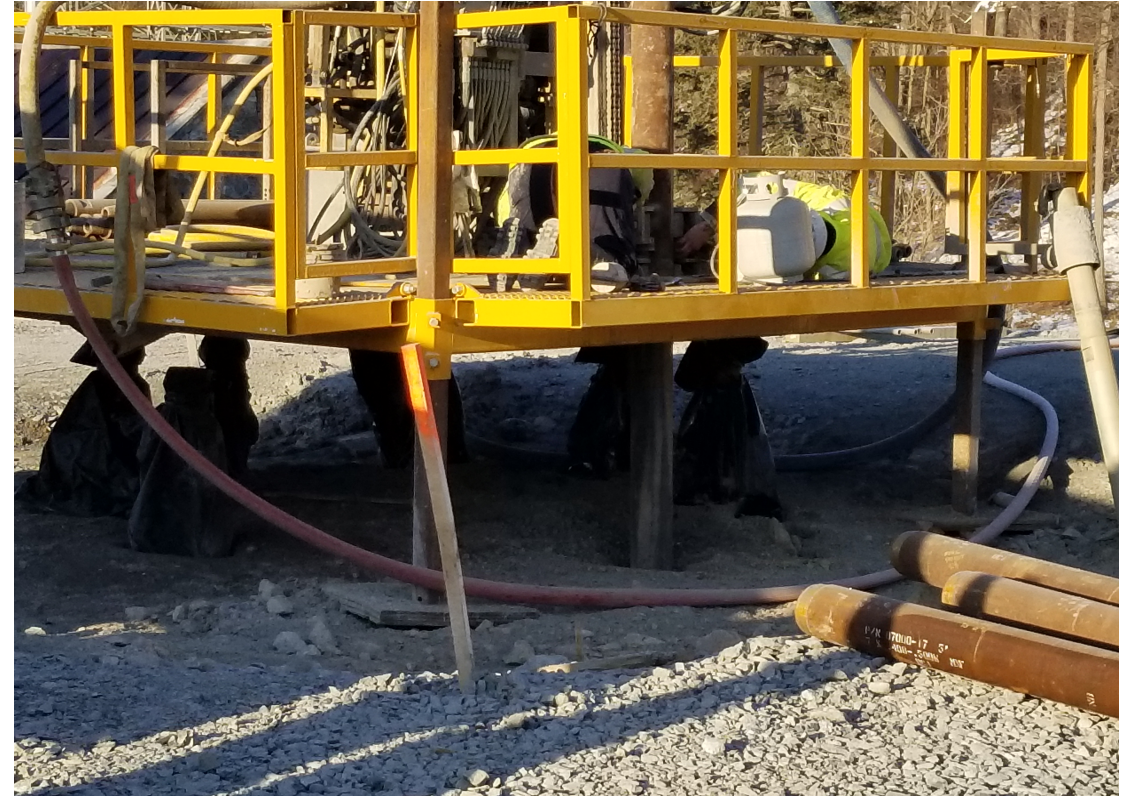
Micro-pile drilling
