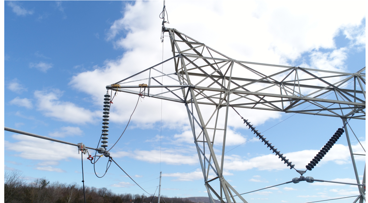
Repaired Structure Arm
