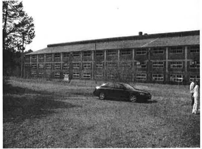
View from the east towards main building
