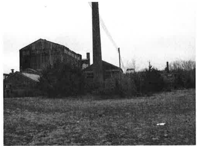
Site buildings viewed from the north
