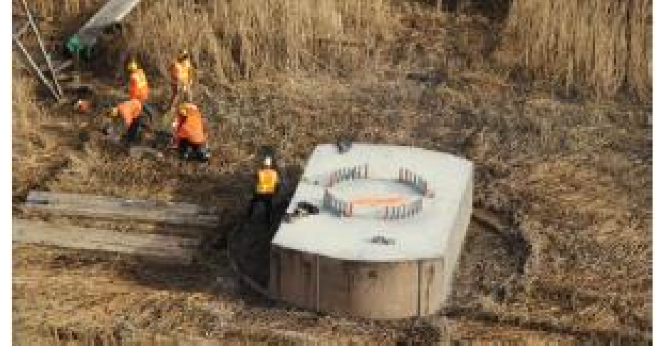
Concrete Pile Cap
