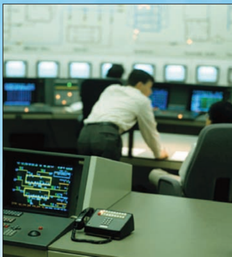
NYISO determines the order in which power plants are dispatched to meet New York's energy demands.
